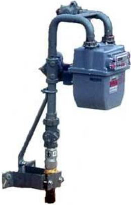
Each natural gas service is equipped with a meter which serves the customer. The meter is owned by the gas company. In an emergency the gas to any house can be shut off at the meter.
