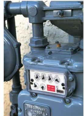
**Do not hang garden hoses or tie dogs to the gas meter piping. The stress may cause the pipe fittings to leak and become hazardous.**
