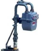
Each natural gas service is equipped with a meter which serves the customer. The meter is owned by the gas company. In an emergency the gas to any house can be shut off at the meter.
