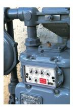
Do not hang garden hoses or tie dogs to the gas meter piping. The stress may cause the pipe fittings to leak and become hazardous.
